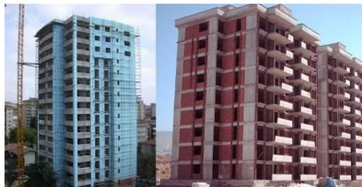
**Figure 1:** Polystyrene based foam used in insulating buildings for thermal effects on a clay brick facade wall on the left and before insulation and plastering on the right.
