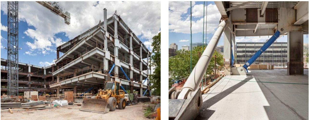
Figure 1 – New construction of the Salt Lake City Public Safety Building, a post-disaster performance level steel moment building frame using fluid viscous dampers (Holmes Culley, San Francisco).
